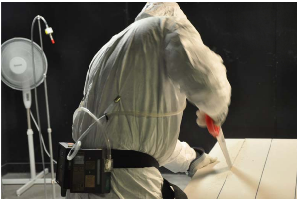
Figure 7. Cutting a 5/8" Type X drywall board section with the hand saw.
