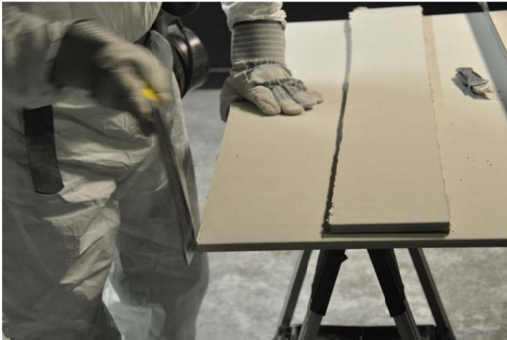
Figure 6. R rasping the rough cut edge of the main drywall board section using the shaping file/forming plane.
