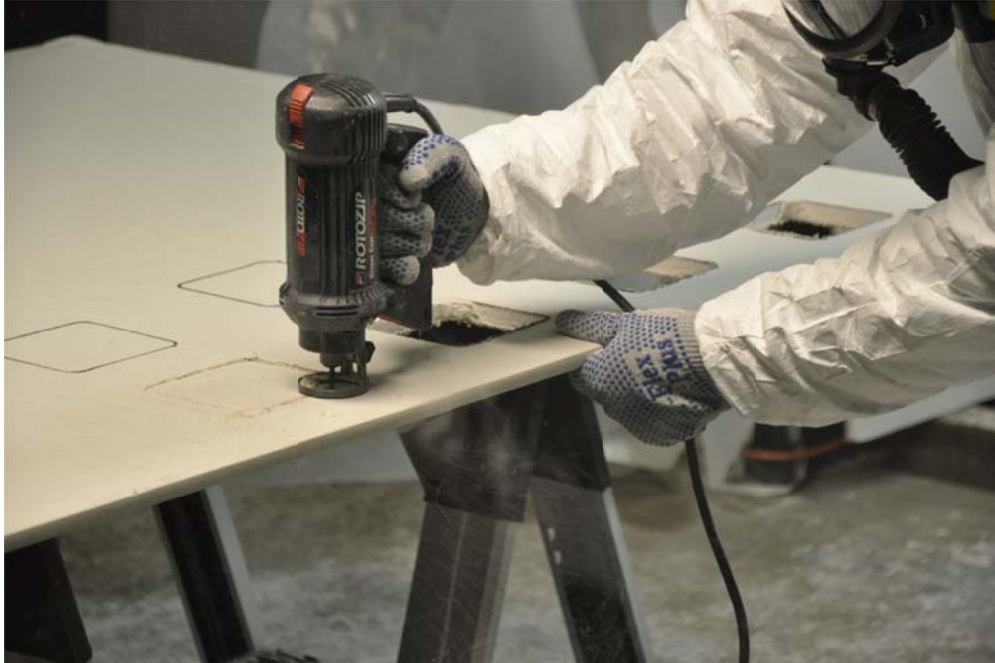
Figure 10. Cutting a 5/8” Type X drywall section with the rotary (i.e. rotozip) saw.
